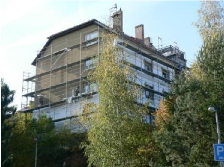
Installation of external insulation to the “Na Stárce” building
